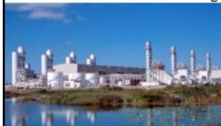
Liquefying air or other gases plant
