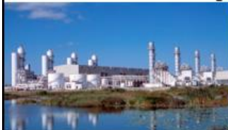
Liquefying air or other gases plant
