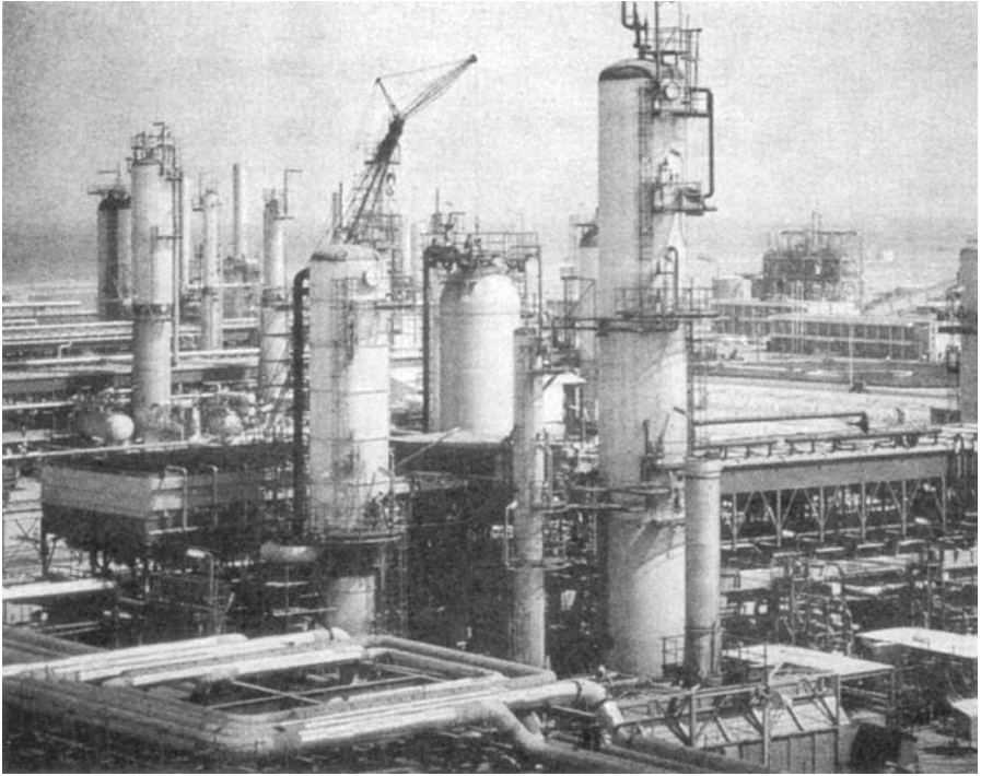
E.11 24,000 BPD H-Oil™ unit. (Photo courtesy of Fluor Engineers and Constructors, Inc.)
