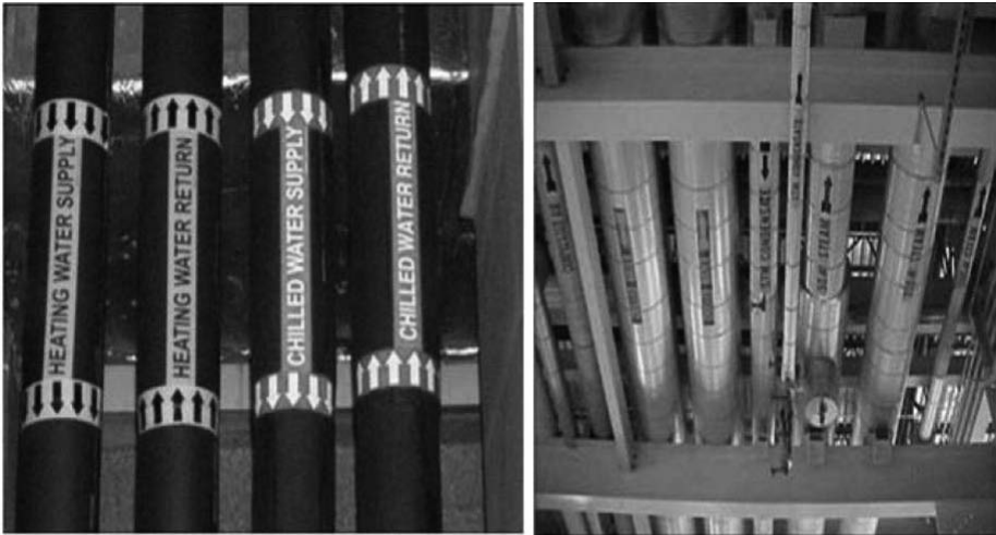
Figure 7.2d Examples of Color-Coded Pipes and Hoses
